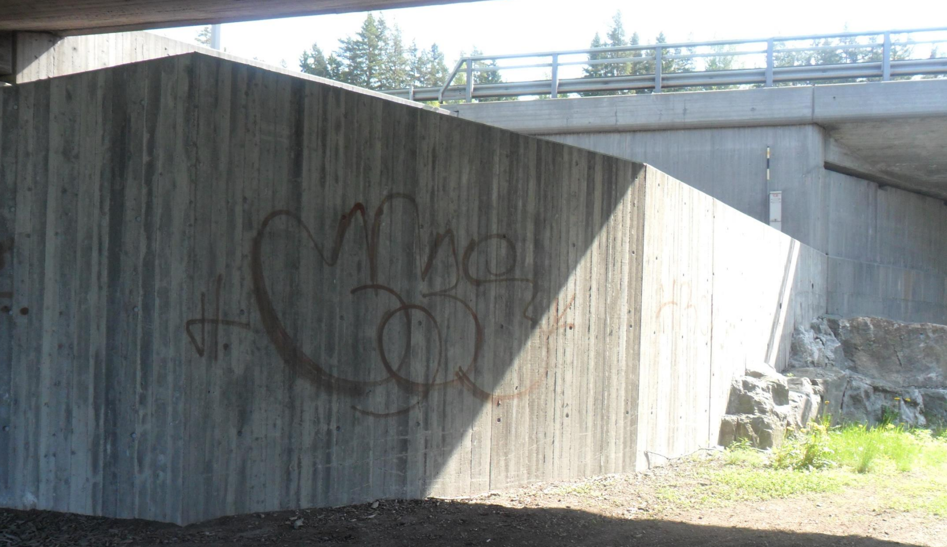
Retaining wall E6 – Taraldrud (built 2004) 100% replacement of coarse aggregates
