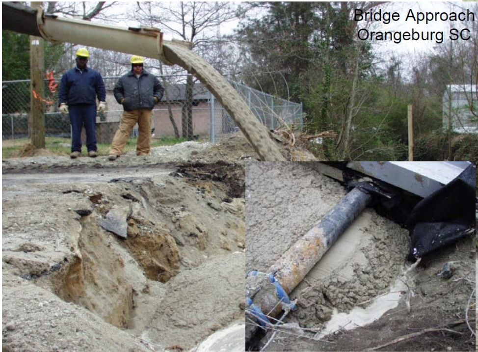
Void Fill Courtesy of Tom Fox
