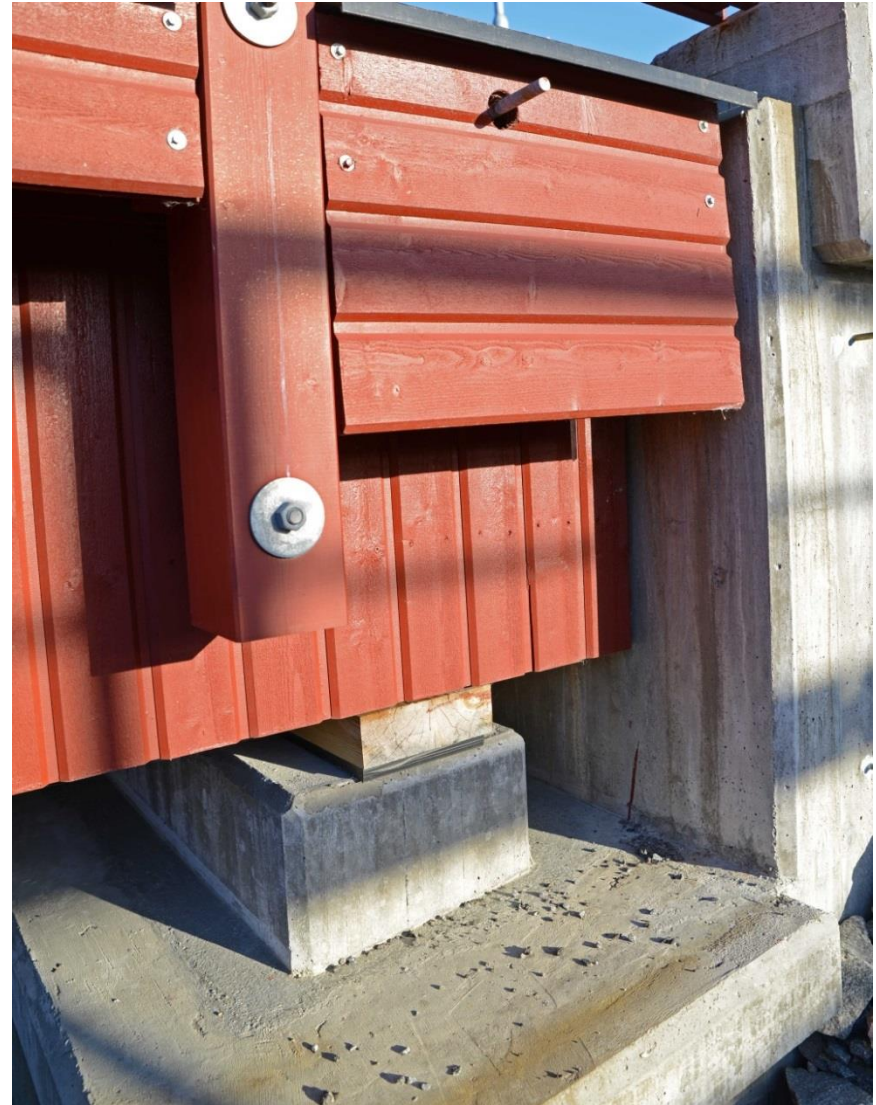
Stackgrönnan bridge 2010, photo P-A Fjellström
