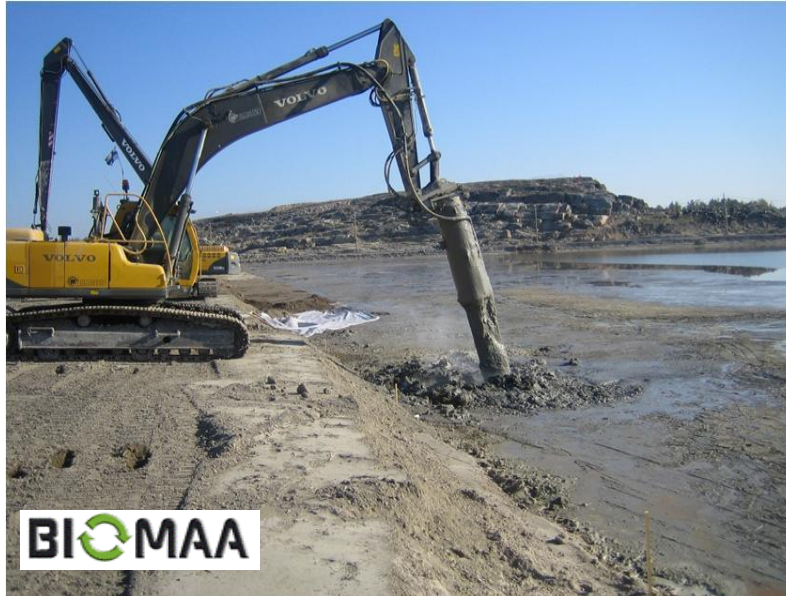
MASS STABILISATION - Stabilisation depth usually 2...6 m
