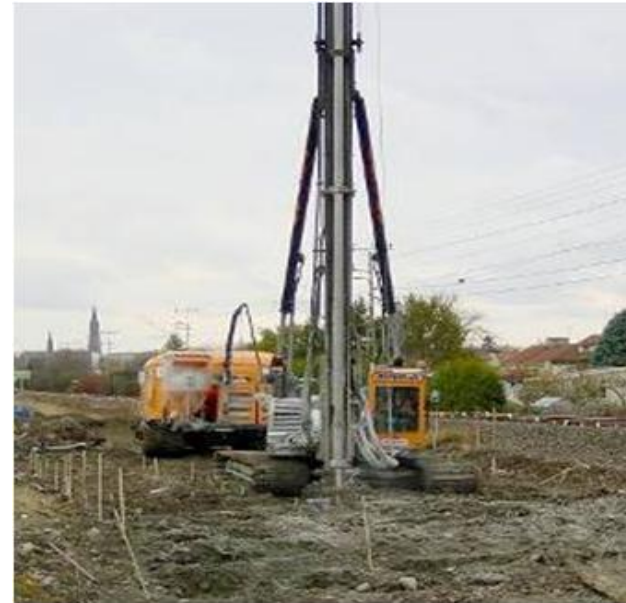
COLUMN STABILISATION - Stabilisation depth usually > 6 m
